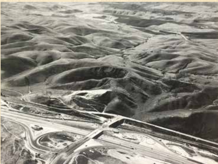
Oso Parkway & 5 Freeway Ziggurat building (at top) construction in progress.
