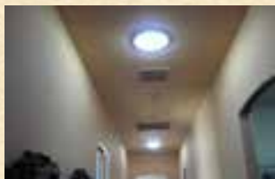
A Solar Tube installation
