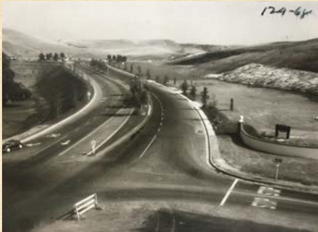
Crown Valley off-ramp
