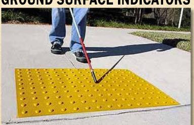
Mission Viejo is installing truncated domes at the base of access ramps on city streets. These are detectable warnings which enable people with visual disabilities to determine the boundary between the sidewalk and street. Because truncated domes have a unique design, they can be detected underfoot and by sound on cane contact.
